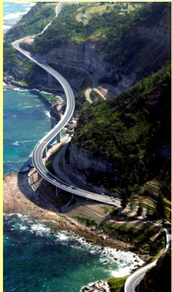
Pacific Coast Highway in Australia. Replacement of one of the most dangerous sections. Existing highway had to remain functional while new highway was built.
